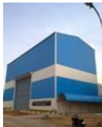
Figure-1 Transformer Repair Bay
